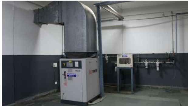
❖ Compressed Air Generation & Distribution System
