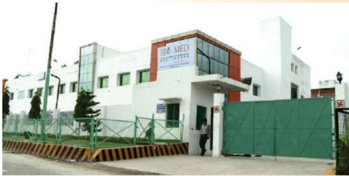
Facility At Sidcul, Haridwar, Uttarakhand
