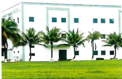
PELLETS AND DC GRANULES PLANT AT VIZAG
