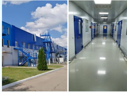
OSD Plant Skidel - Belarus
